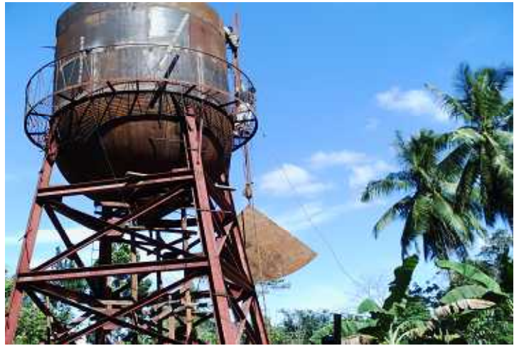
Contractor welders are lifting a section of top cover for installation
